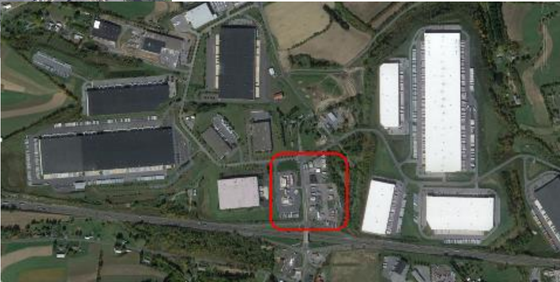
Sheetz and Onvo Stores in New Smithville, PA (I-78)
