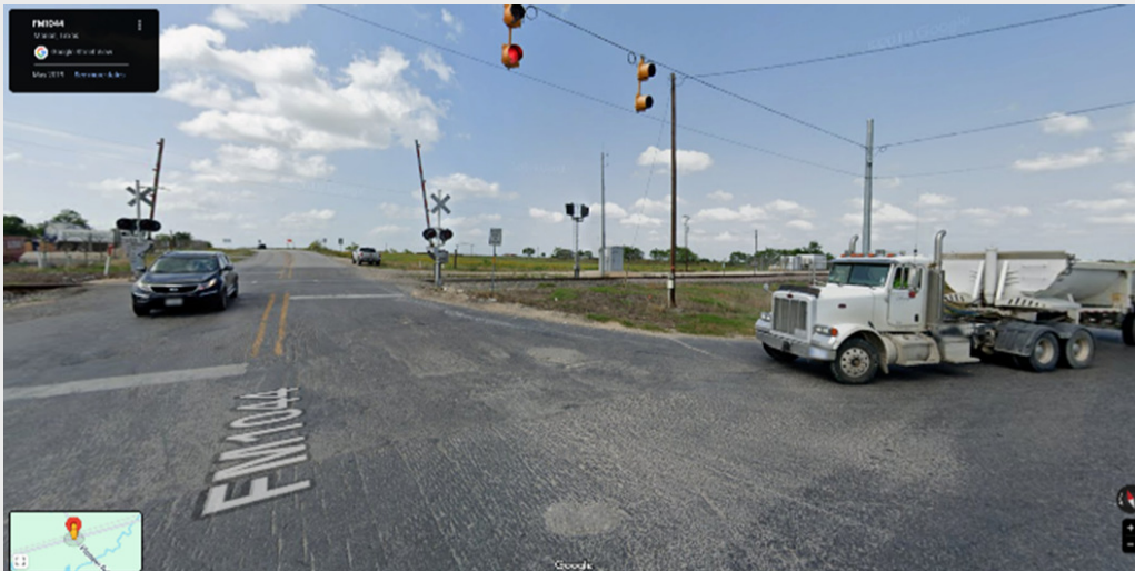
Looking northbound on FM 1044. Note the close proximity of the RR crossing to the intersection.
