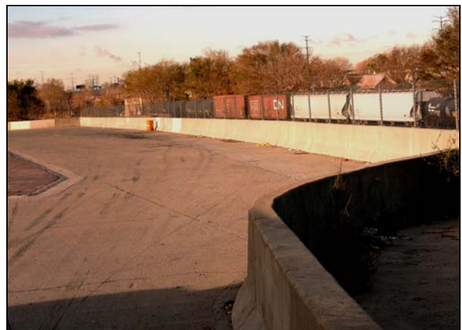
Throop Street AIS, Stevenson Expressway Chicago, Illinois AIS located off Mainline
