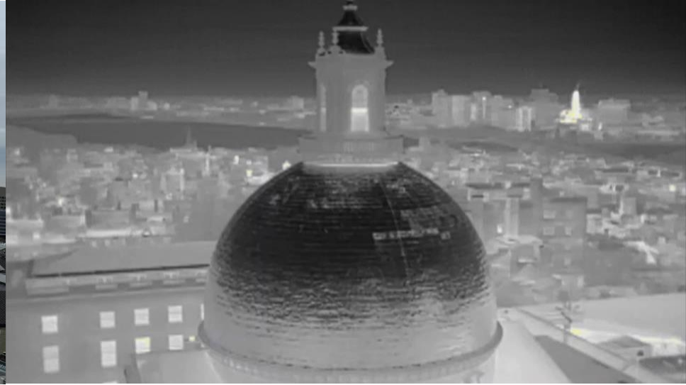
IR imagery of damage
