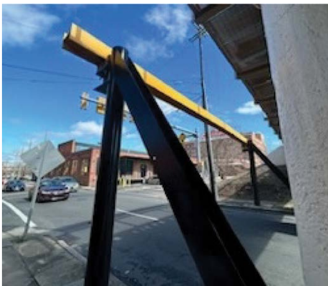
Figure 34. Portal frame (Source: VHB).
