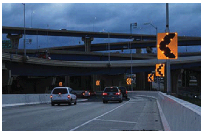
Figure 27. Example of flashing chevron signs on a bridge structure with a horizontal curve (Source: Albin et al. 2016).
